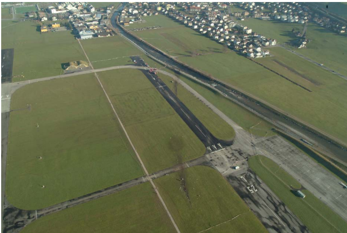
Overview in direction east
