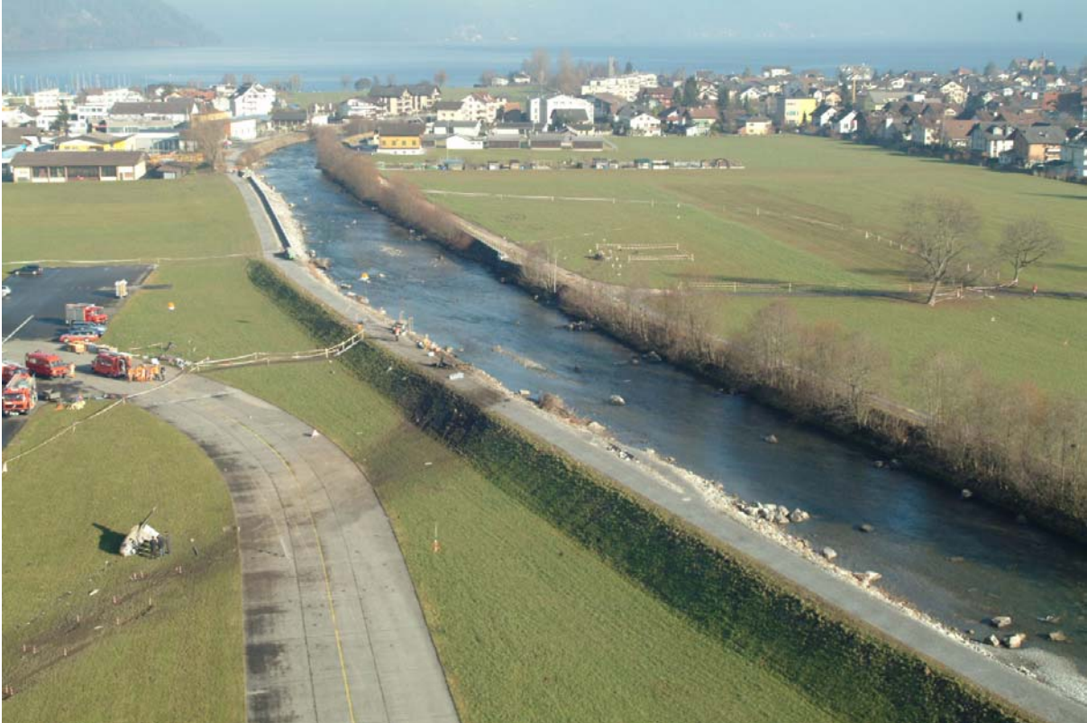
Tail and point of impact on the dam; behind the cockpit in the area of Buochs
